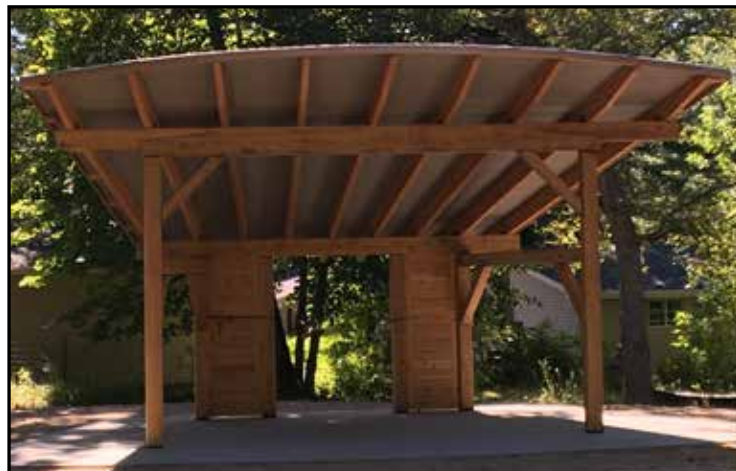
This front view displays the wood side panels that can be slid to the center when the electrical panel is in use.
