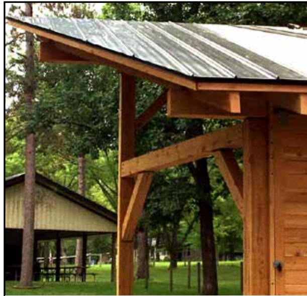
The metal roof was installed during the second week of September.
